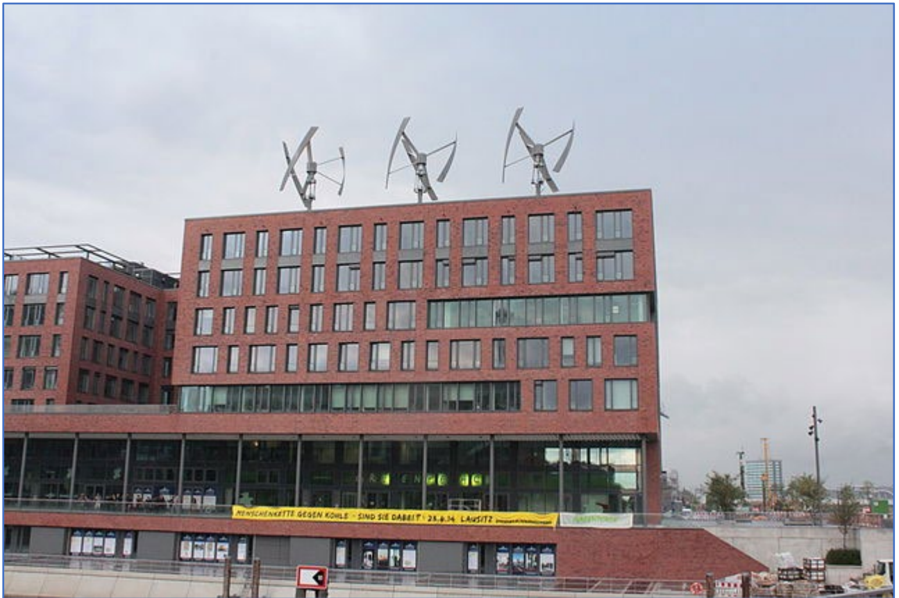
Figure 8: Urban Wind Turbines at Greenpeace offices, Hamburg, Germany
