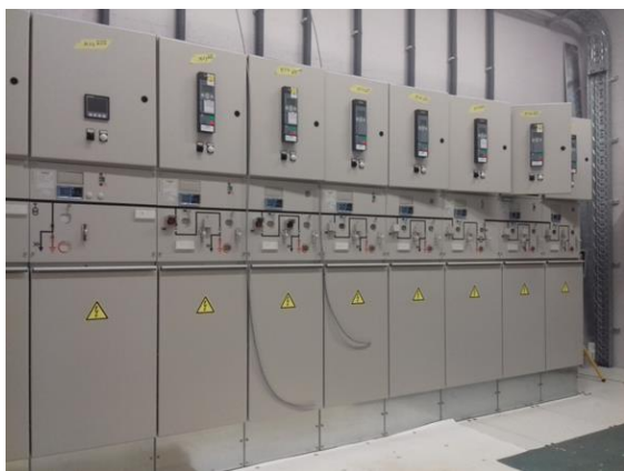
Figure 10 – 3kV distribution board in the new power station South
