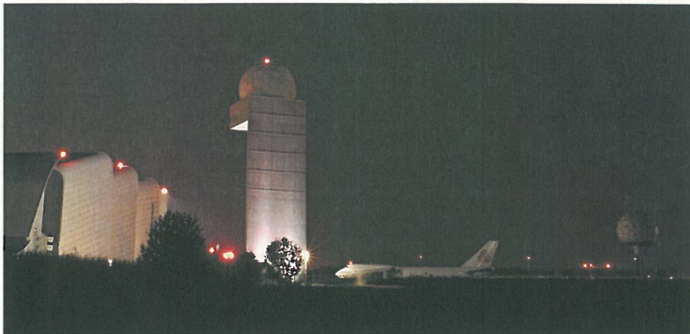
Figure 9 - Terminal radars TAR1 / TAR2 and Cargolux hangar
