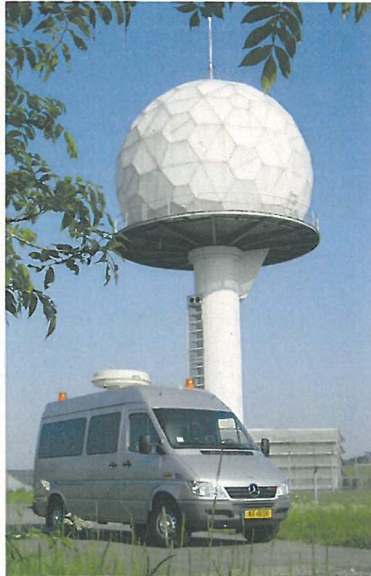
Figure 8 – TAR 1 at Luxembourg Airport
